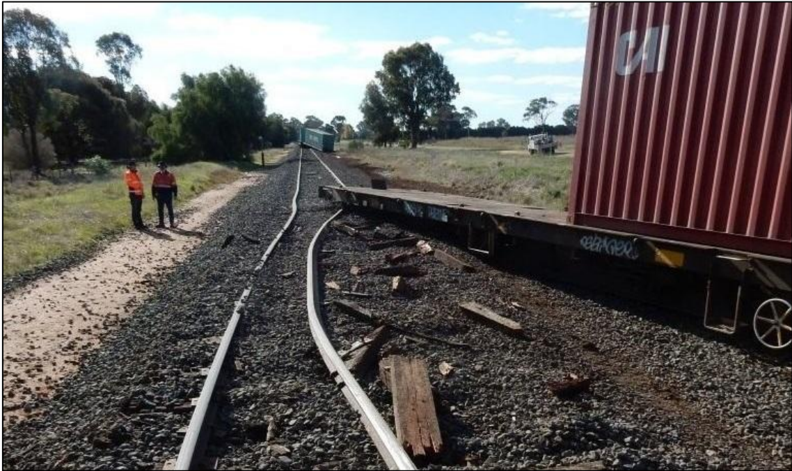
Figure 3: Separated section of train and track damage, looking towards Tocumwal
