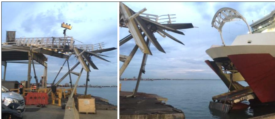
Figure 5: Spirit of Tasmania II 's damaged upper bow ramp (skybridge)
