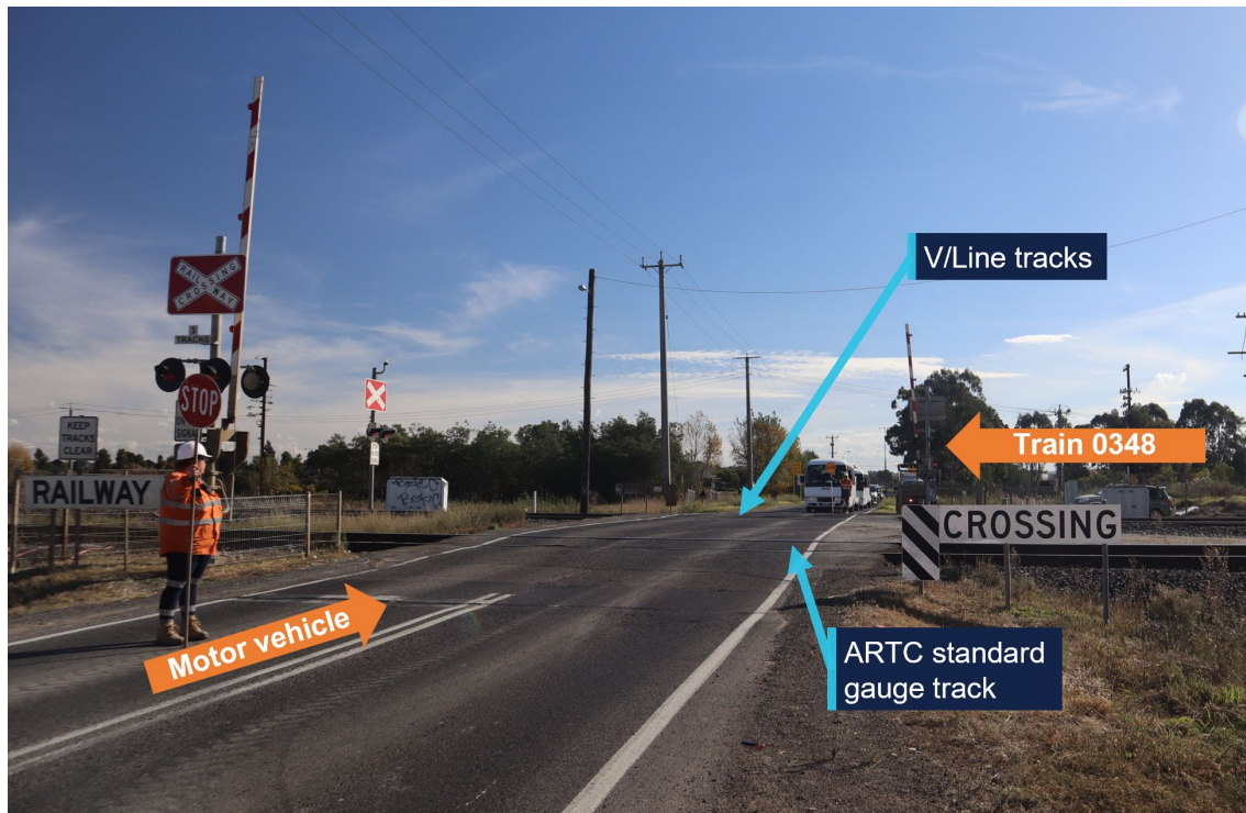
Figure 7: Wallan–Whittlesea Road level crossing, looking west
