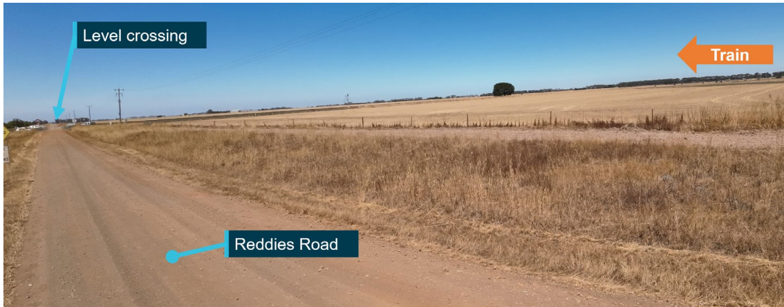
Figure 8: Sighting to the west on approach to the level crossing from the north
