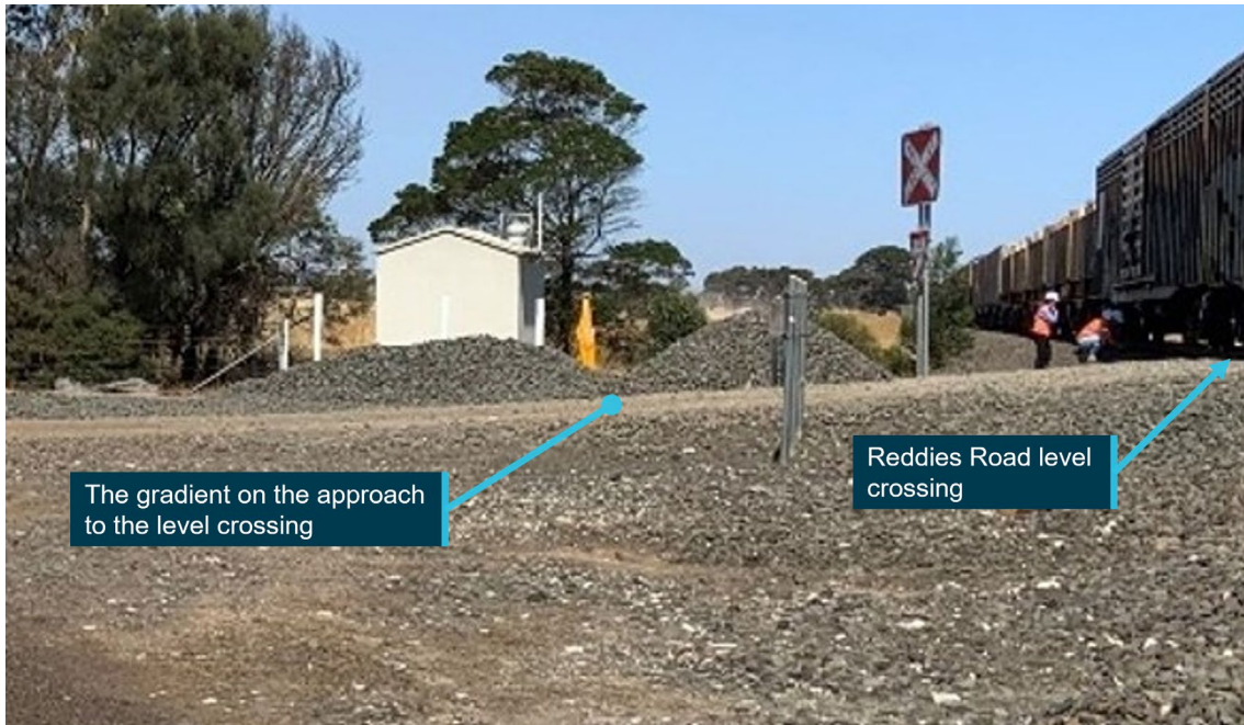
Figure 3: The gradient on approach to the level crossing from the north
