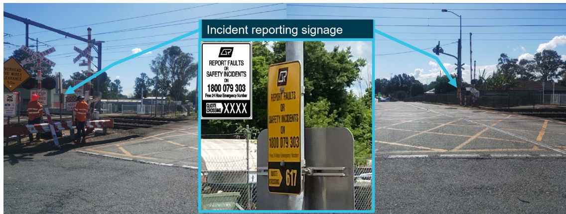
Figure 6: Bonemill Road level crossing incident reporting signage
