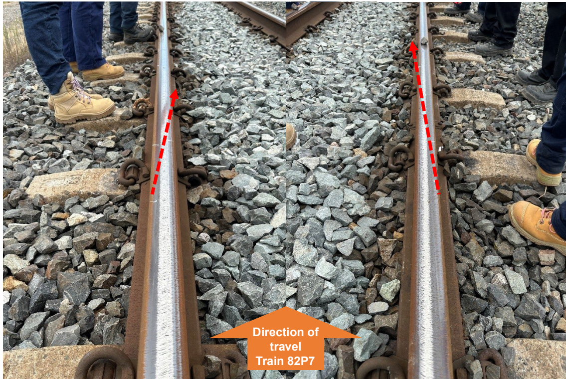
Figure 5: Wheel marks identified on the left and right rail head at the point of derailment
