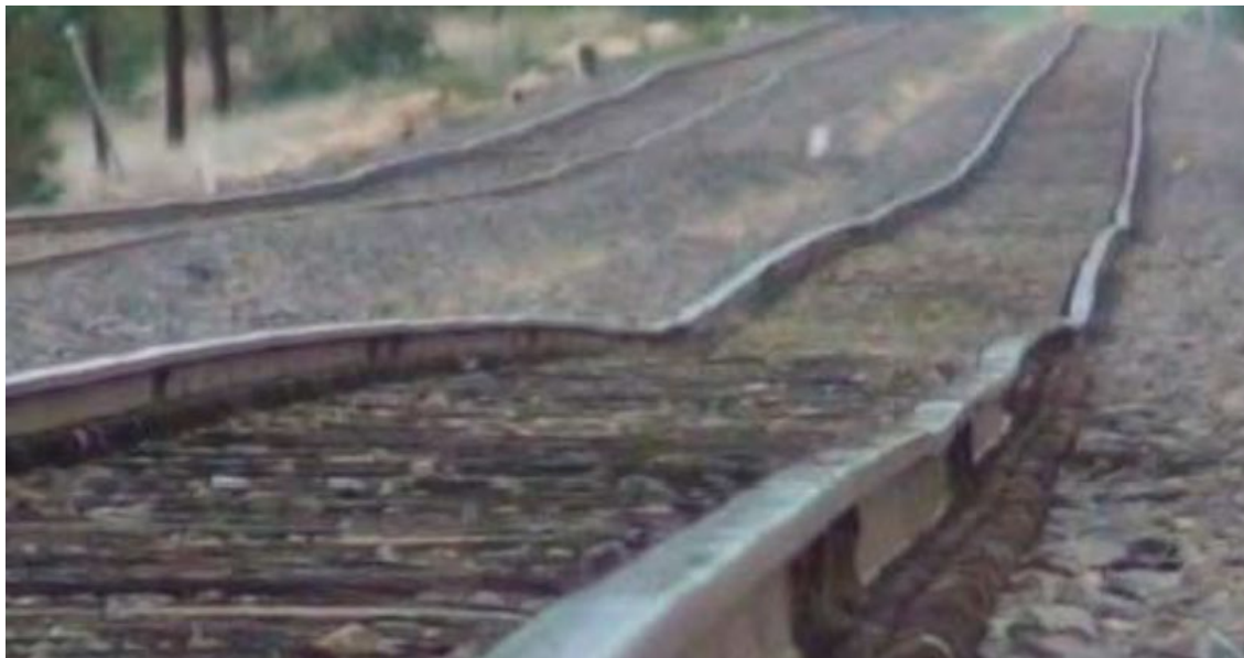
Figure 8: Example – soft formation mud hole
