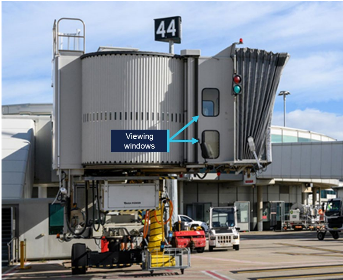
Figure 10: Right side windows on aerobridge at Gate 44 of the Brisbane Domestic terminal
