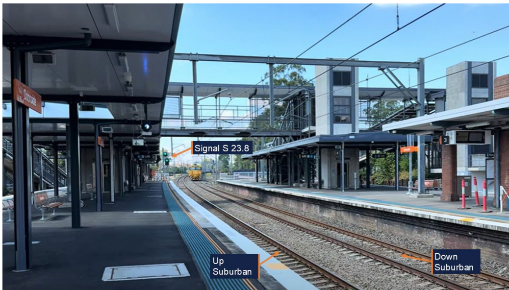
Image from Doonside platform upgrade VLOG. Source: Sydney Trains, annotated by OTSI
