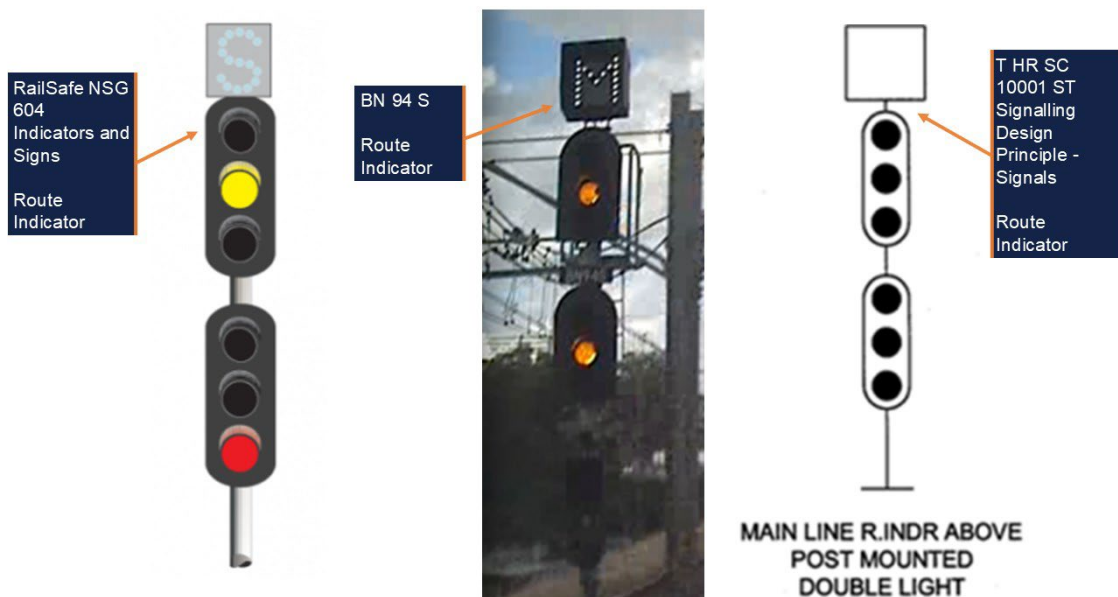
Left: NSG 604 Route Indicator; Middle: BN 94 S; Right: T HR SC 10001 ST Route Indicator. Source: Transport for NSW and RailSafe, annotated by OTSI
