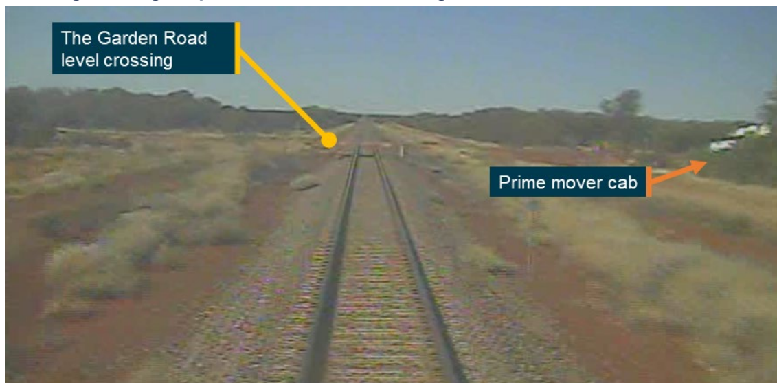
Figure 3: Field of view from the locomotive camera approximately 120 m from the level crossing showing the prime mover cab as it emerged
