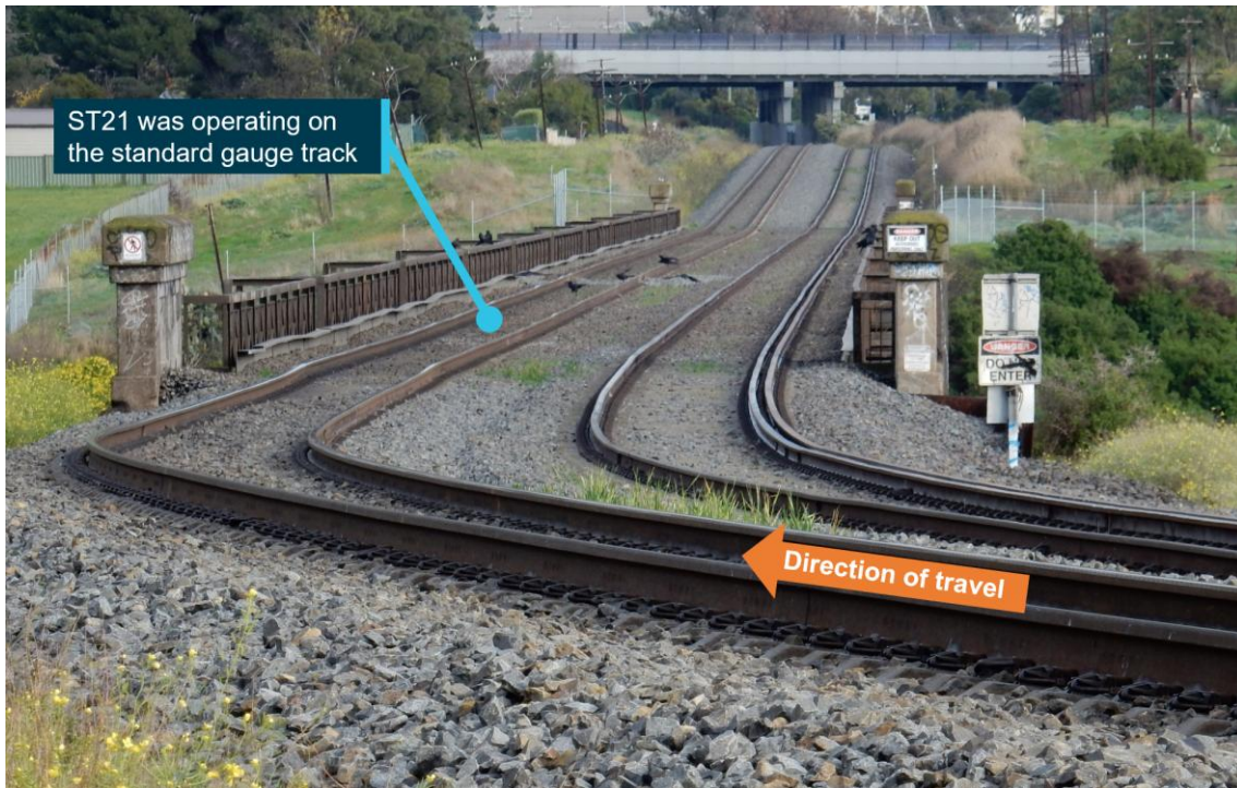
Figure 5: The location of the TSR at the Moonee Ponds Creek Bridge
