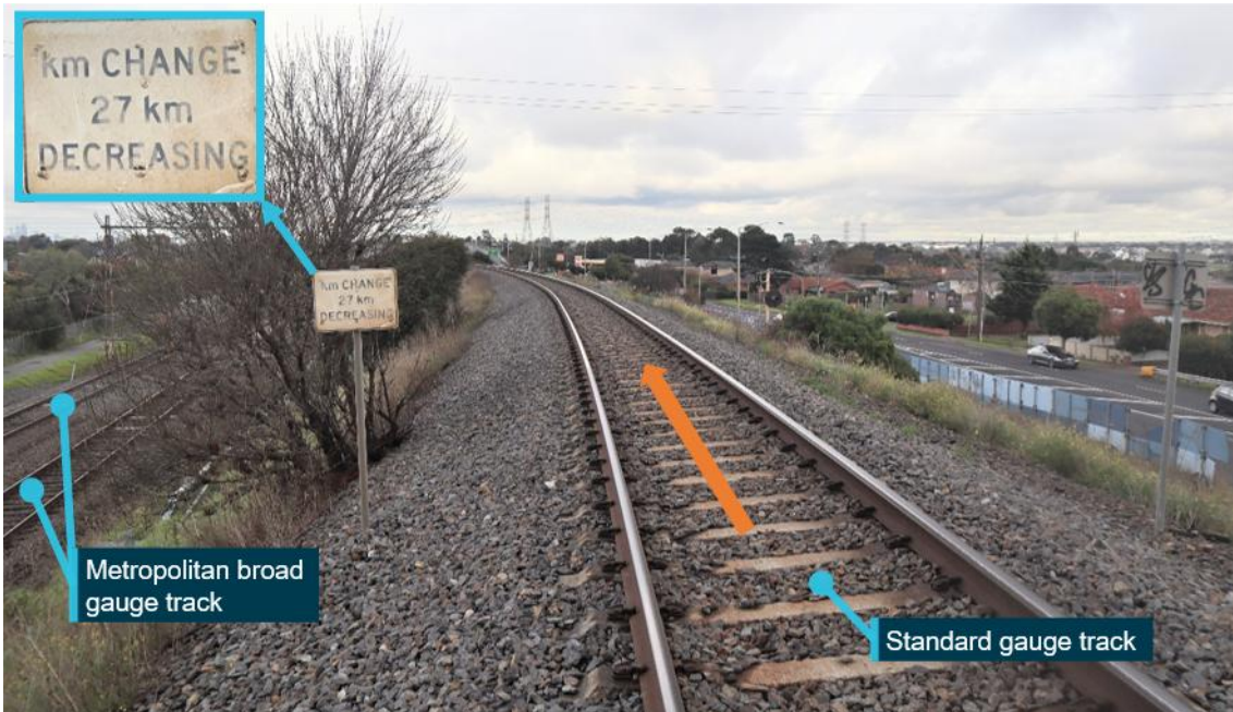
Figure 4: Kilometre change notification on the standard gauge track at Jacana flyover
