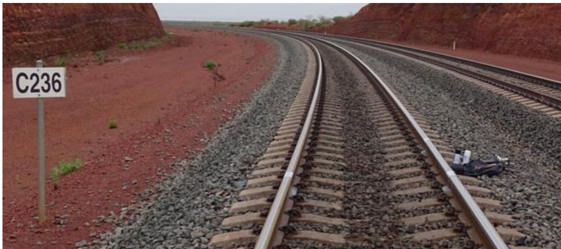
Figure 9: An example location marked using the ‘C’ prefix on an Australian railway
