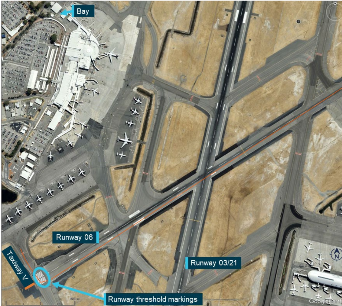
Taxi and take-off roll during the departure is shown in orange. Source: Google Earth, annotated by the ATSB
