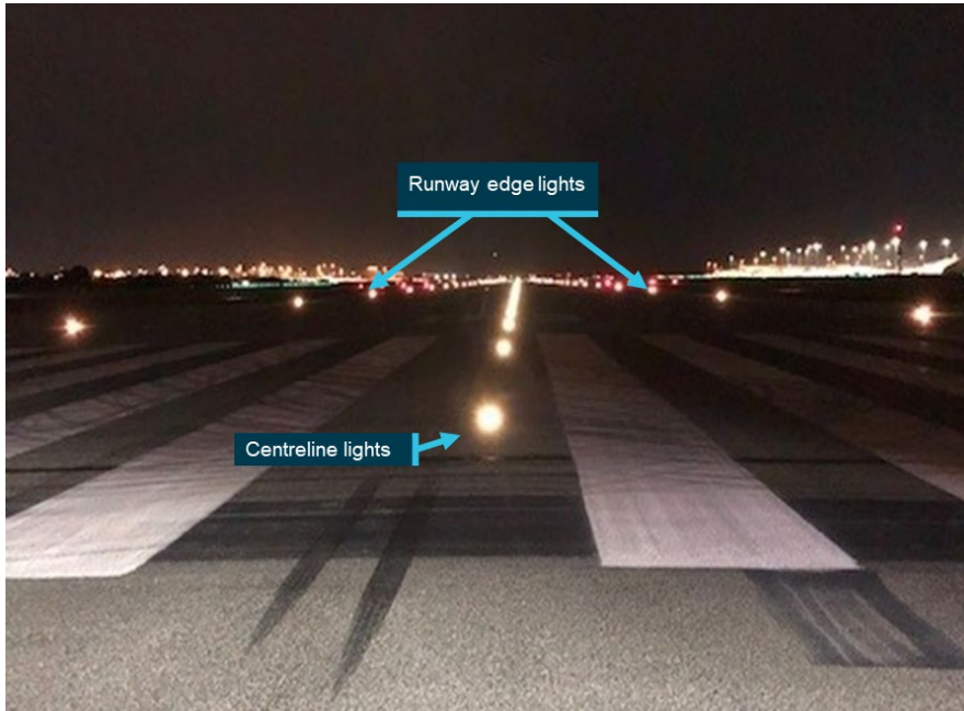
Figure 6: Runway centreline lights and edge lights on runway 03
