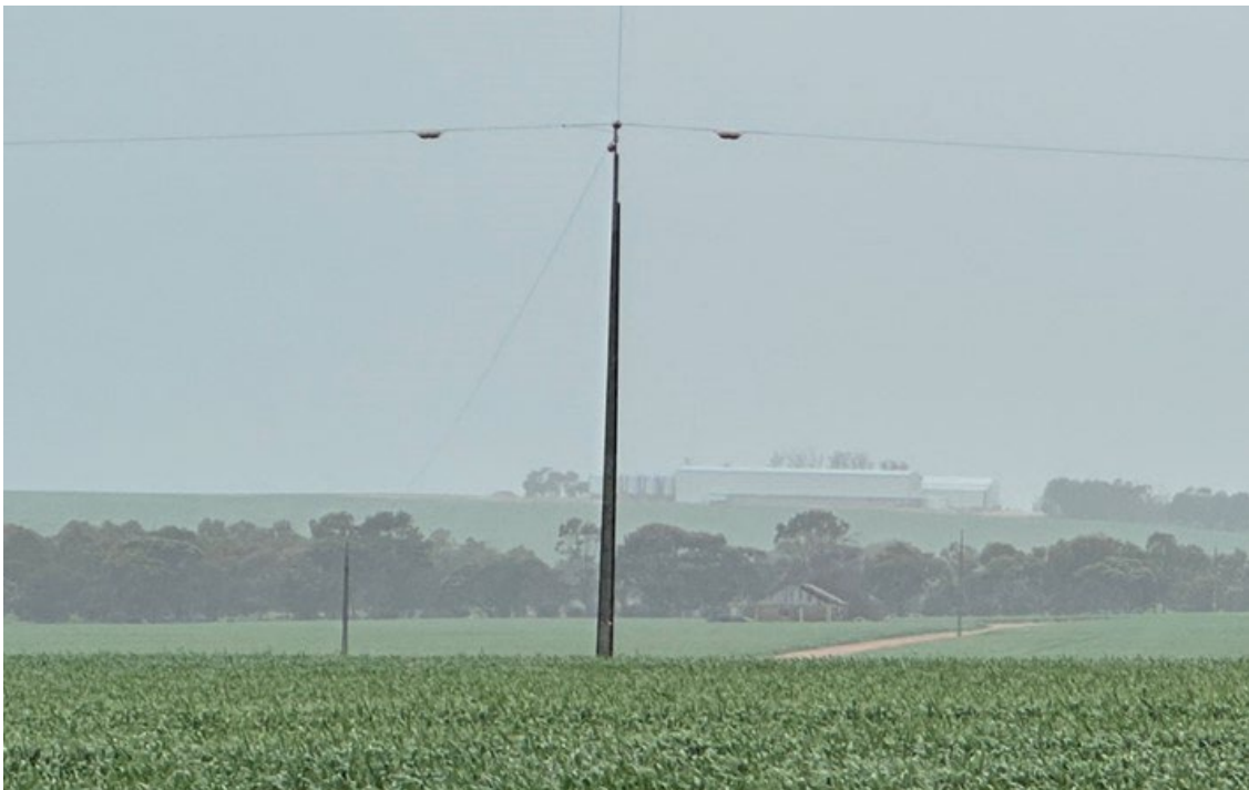
Figure 2: 19 kV single-wire earth return powerline in one of the fields being sprayed
