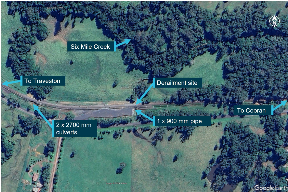
Figure 9: Cross-track drainage systems installed near the derailment site
