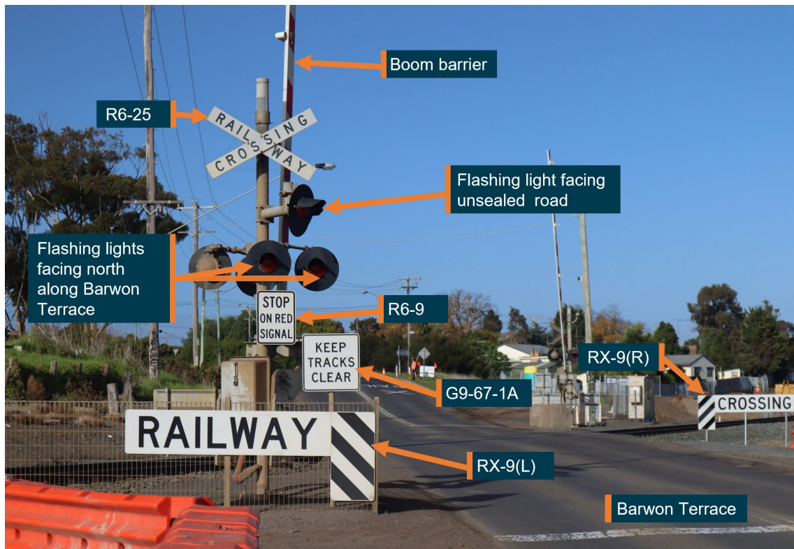
The figure shows the protection equipment at the level crossing on the western side of the crossing. Source: The Office of the Chief Investigator
