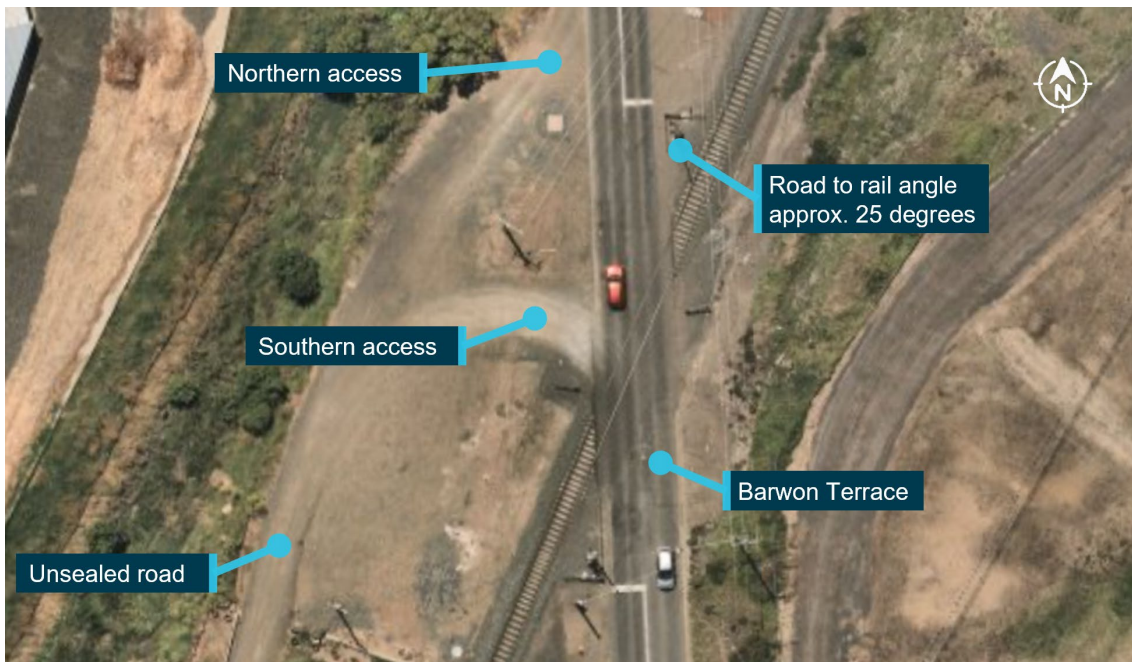
Figure 3: Barwon Terrace interface with rail line
