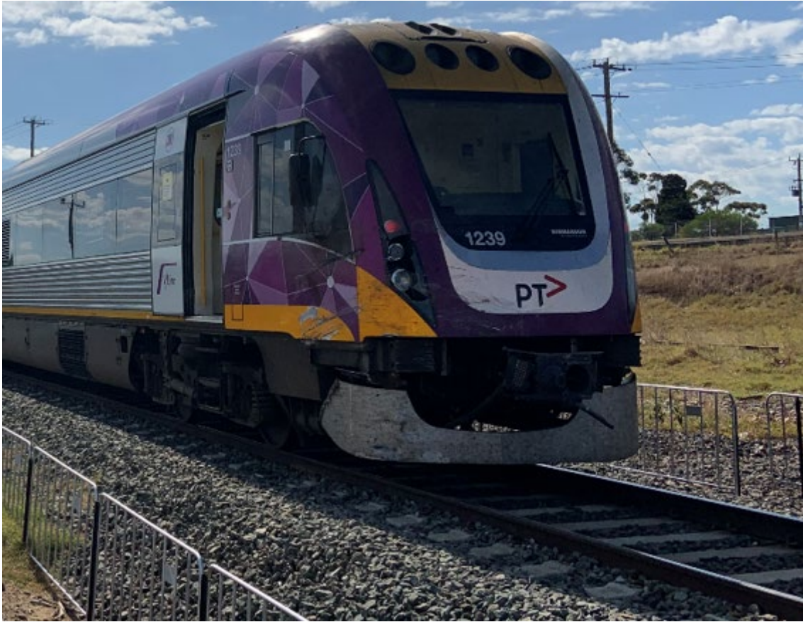
The damage to the front of VLocity train 7727 following the incident. Source: The Office of the Chief Investigator
