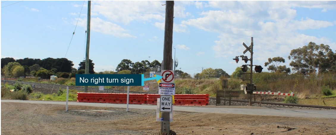
Photograph showing the no right turn sign on the power pole. Source: The Office of the Chief Investigator
