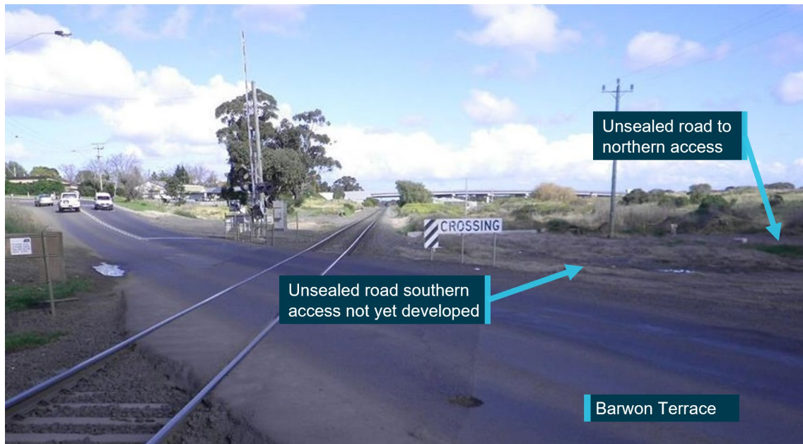
Figure 5: Junction between the access road and Barwon Terrace in 2017
