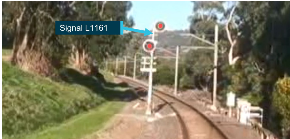
Figure 3: Signal L1161 on the approach from FTG, annotated to show at stop
