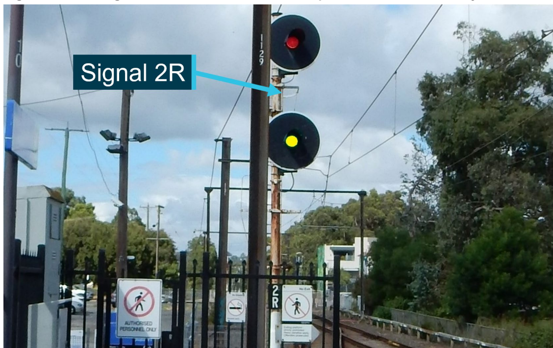
Figure 3: Home signal 2R located at the end of the platform at Ferntree Gully station
