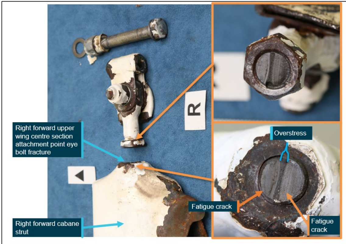
Figure A2: Right cabane strut forward upper wing attachment eye bolt showing evidence of significant fatigue cracking through the threaded portion (Detail A from Figure A1)
