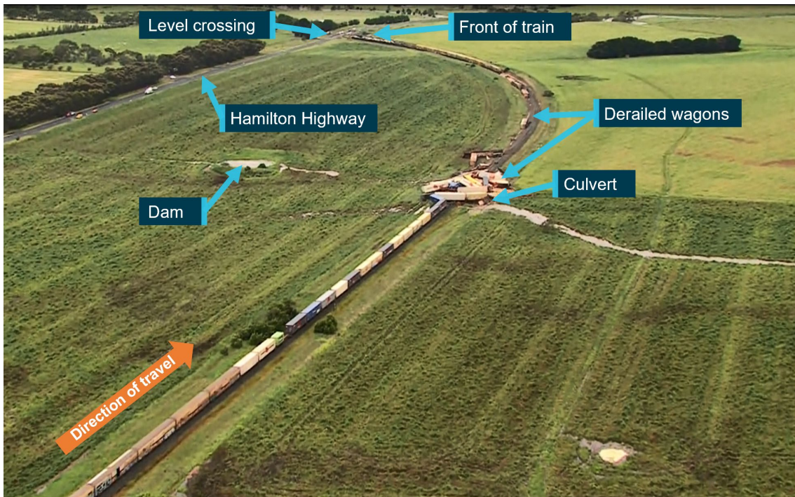
Figure 2: Aerial view of derailed train 4PM9
