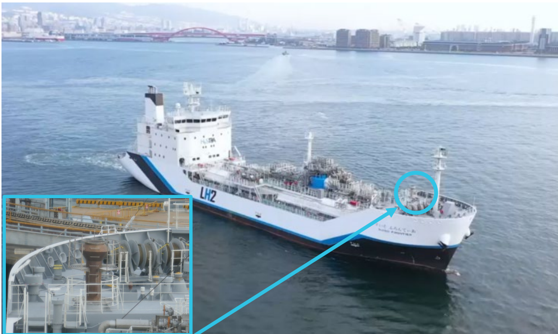
Figure 2: Location of the GCU vent stack
