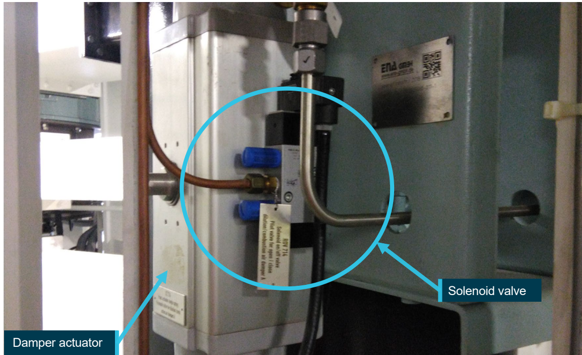
Figure 4: The vent damper actuator solenoid valve
