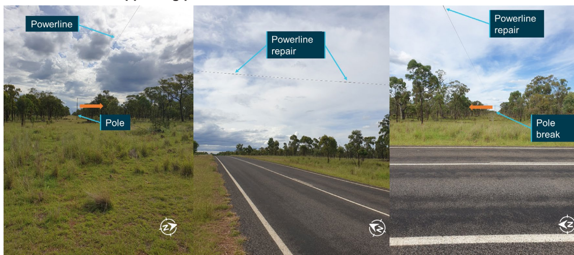
Figure 3: Powerline above the Kennedy Developmental Road showing location of break and direction of supporting pole movement
