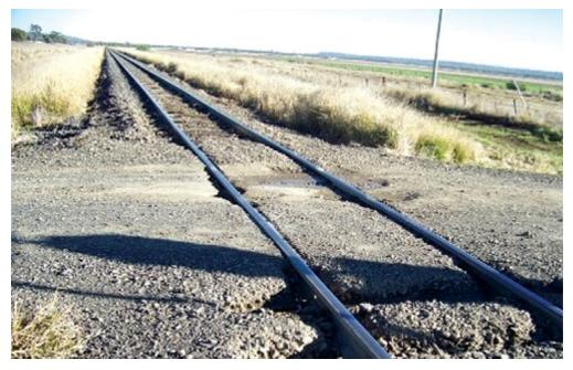
Source: QR. The assessors report recorded that the crossing gravel surface is breaking up and the track is 'pumping' and contributing to surface deterioration.
