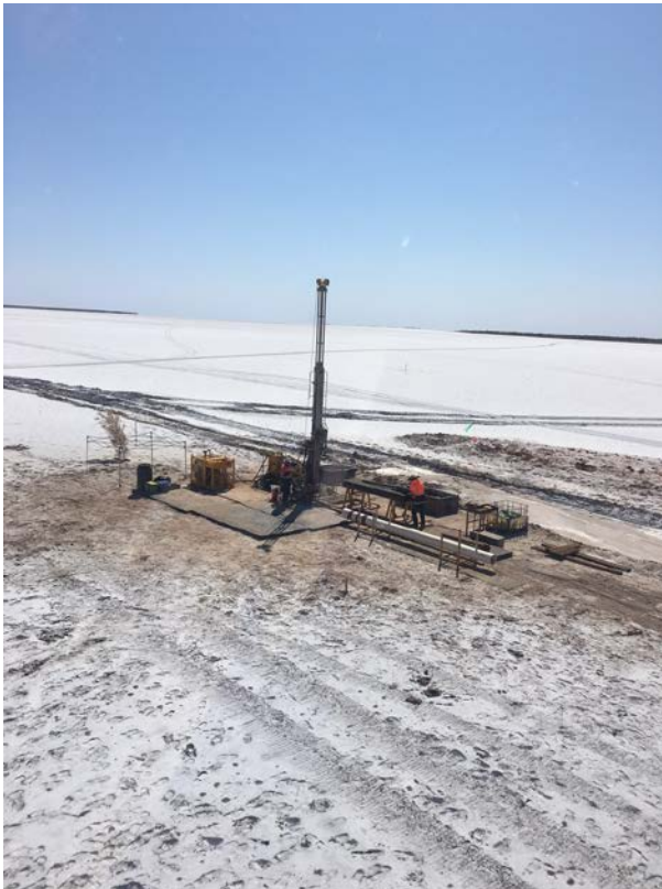
Figure 1: Drilling rig on Lake Disappointment
