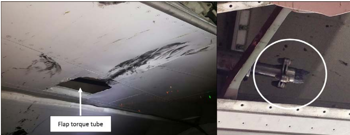
Figure 5: Punctured panel (left) and broken flap torque tube (right) (panel removed)
