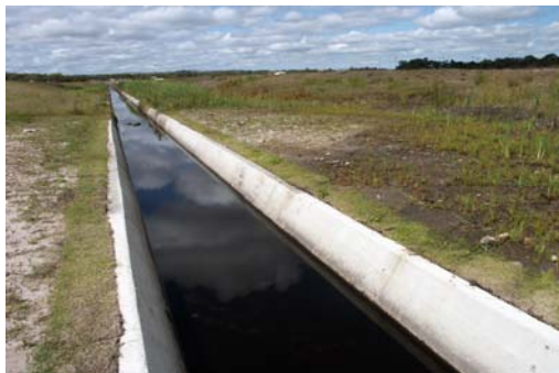
Steep-sided drains, Sunshine Coast Airport
