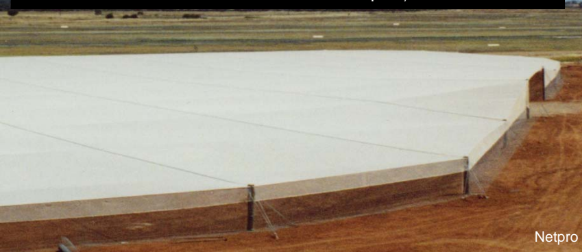
A net used to exclude birds at Parafield Airport, South Australia
