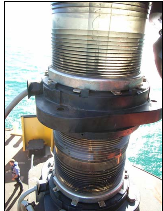
Figure 5: Forward anchor lights
