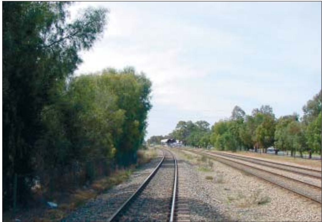
FIGURE 3: Rail approach to Park Terrace
