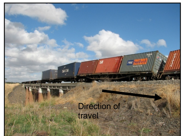
Figure 1: Point of derailment on bridge
