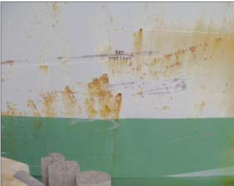
FIGURE 7: Starboard bow of Silver Bin , showing damage to paintwork at point of impact.
